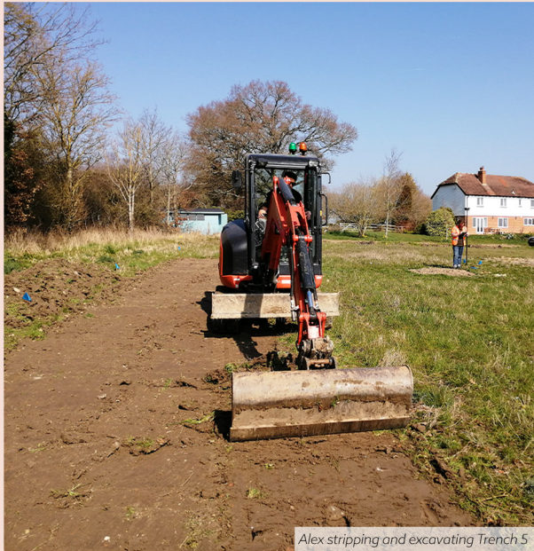
Alex stripping and excavating Trench 5
